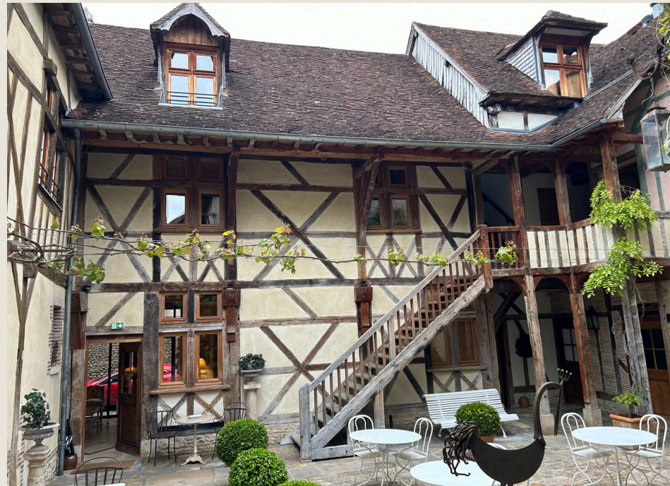
Initial state of the roof
