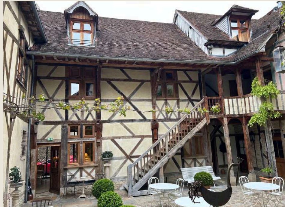
Initial state of the roof
